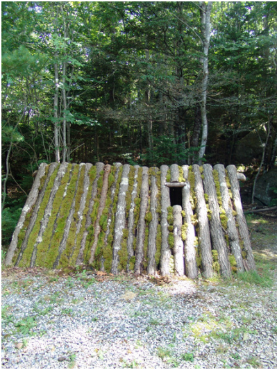
A "pit hut" that was home to the black loyalists during their stay in Nova Scotia. This was nothing more than a log roof over a small pit in the ground. Try to imagine a Nova Scotian winter in one of these.
